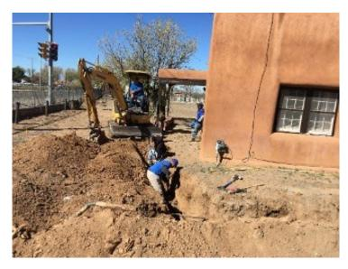
Approximately 75 feet of new pipe was laid, in addition to approximately 90 feet of pipe being re-lined with the latest epoxy resin material. This project remediated a failing sewer pipe and included installing a check valve and two new sets of clean-outs. Some work under the residence still needs to be done, but this extensive project should last for many years.
